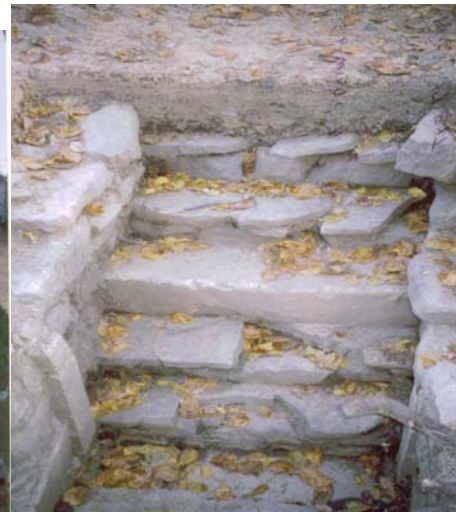
Steps into Historic Foundation
