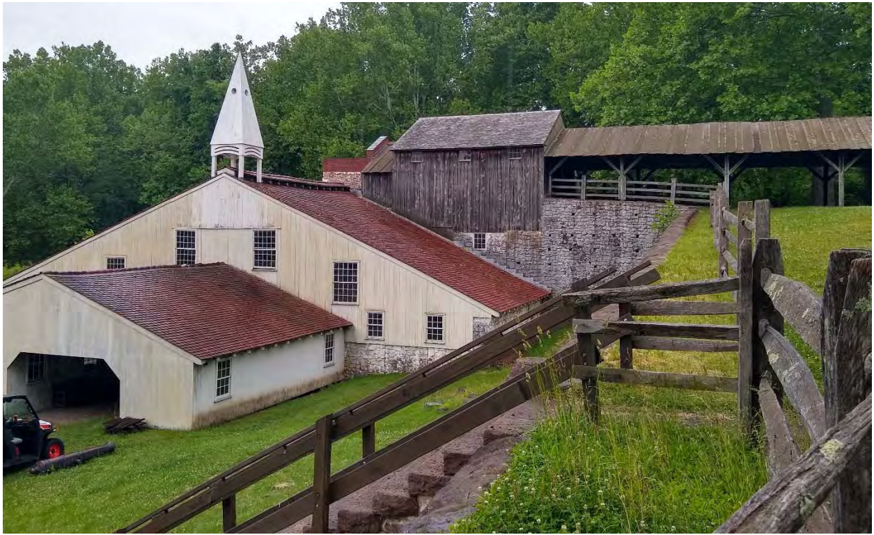
Different view of furnace, casting house, charcoal house and covered way.
