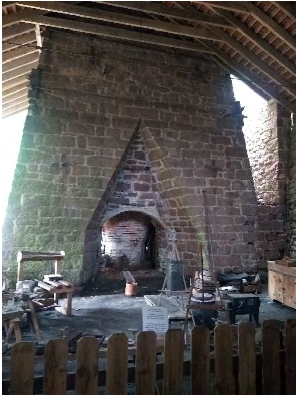
Inside the casting house with the furnace in the background.
