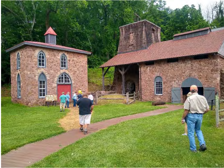
The furnace and casting house and the office building/store have been restored.
