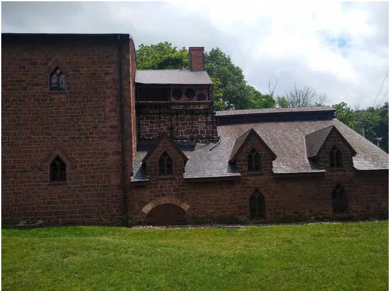
Exterior of Furnace complex and casting house. Note the furnace chimney in the background.
