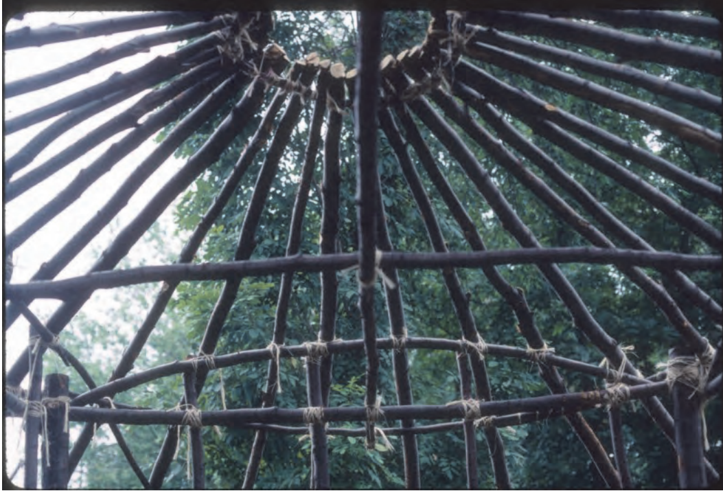
Figure 3. Interior view of parabolic support system and bracings.
