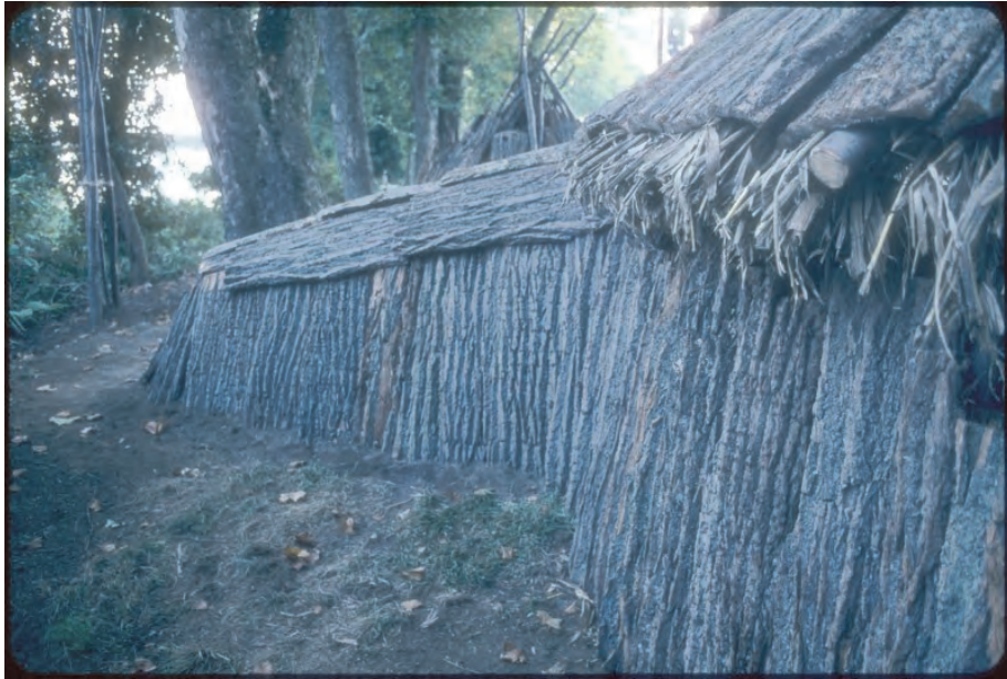
Figure 7. Side view of semi-subterranean appendage with bark cover.
