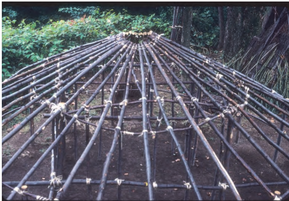
Figure 2. Exterior view of conical roof frame with its parabolic support system.
